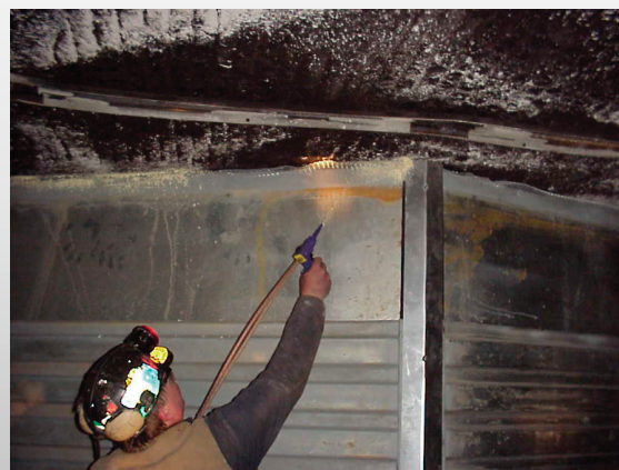
SEAL METAL STOPPINGS
